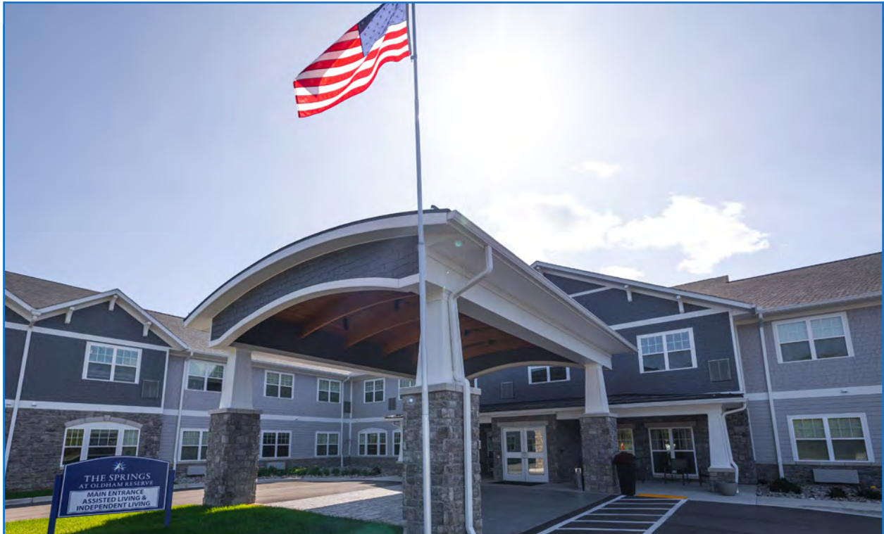
The Springs at Oldham Reserve, a Trilogy Health Services assisted living community. Photo courtesy of Trilogy Health Services.
